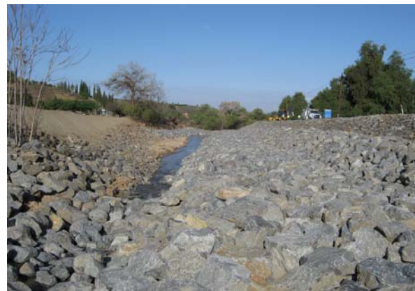
Repair completed in February 2011
