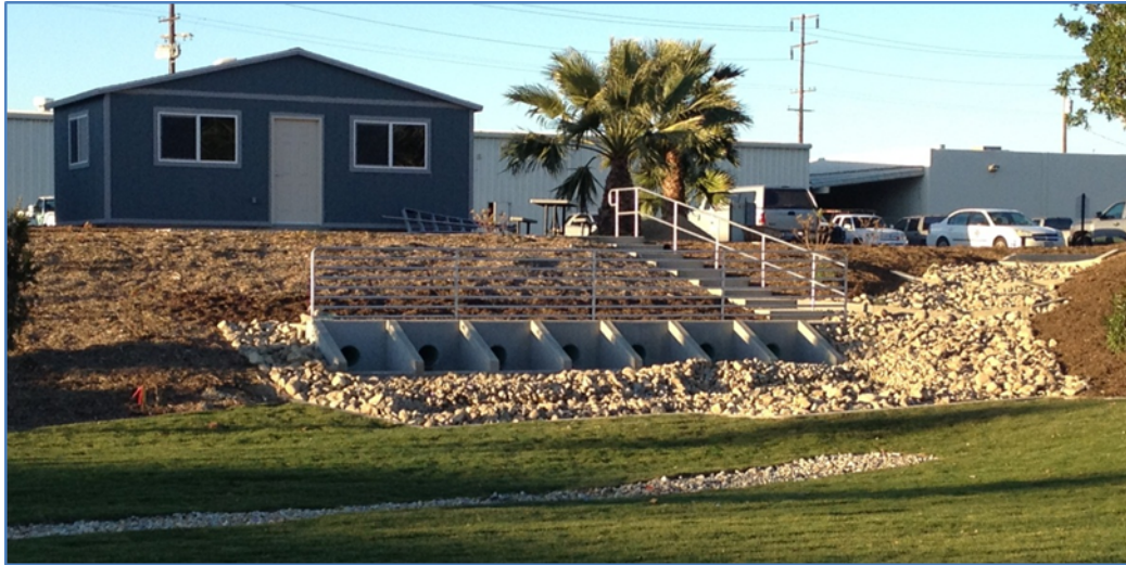
Centralized Monitoring Point for Low Impact Demonstration Project
